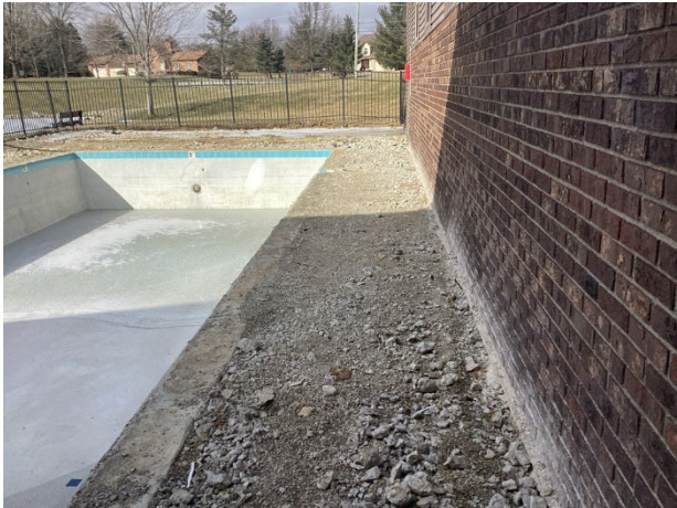
Deck in process of replacement
