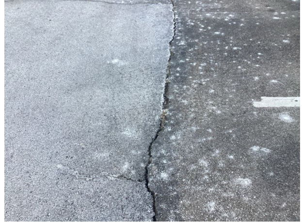
Pavement cracks
