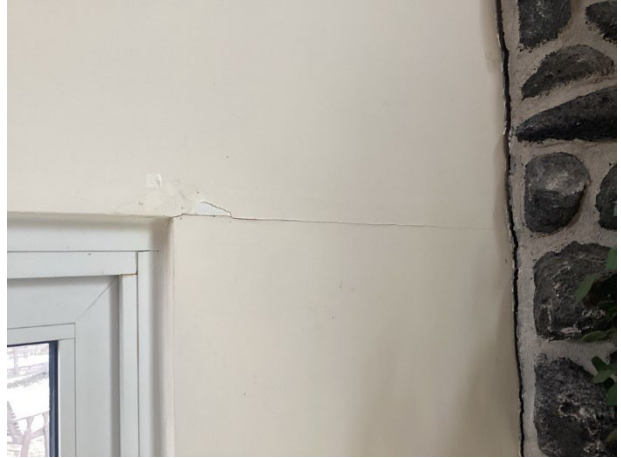
Wall cracks
