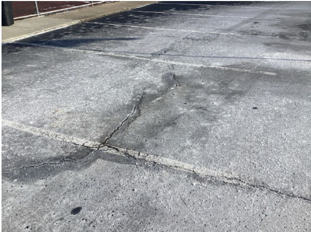
Pavement cracks
