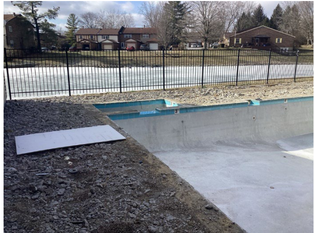
Deck in process of replacement
