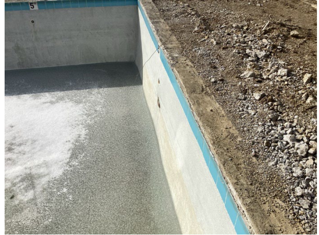
Pool plaster finish with tile perimeter
