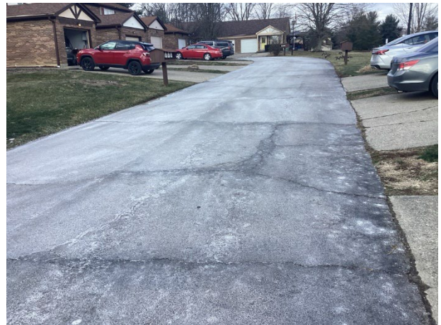
Pavement cracks
