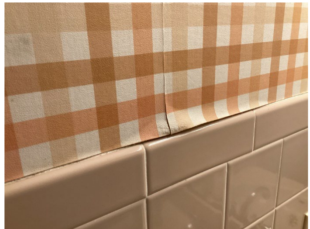
Adhesion failure
