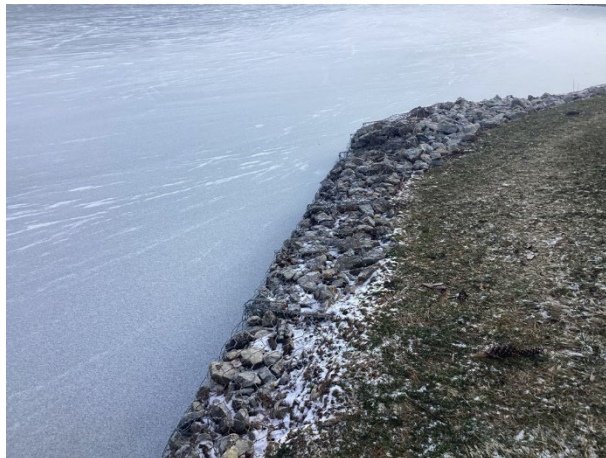
Installation of a gabion wall to forestall erosion near building
