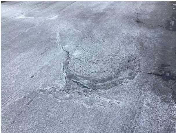
Slippage cracks
