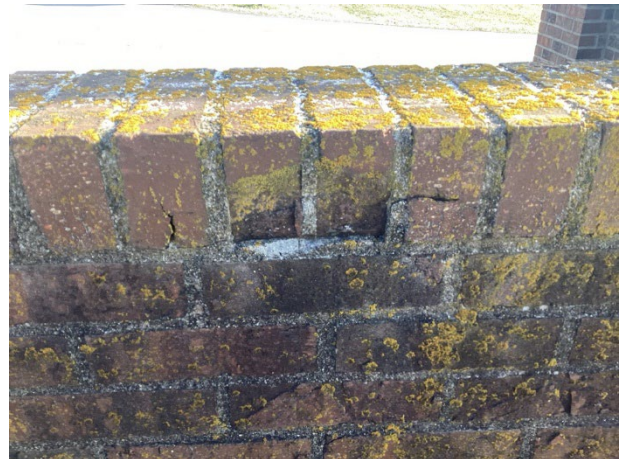
Masonry spall
