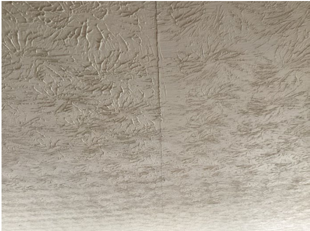
Ceiling crack
