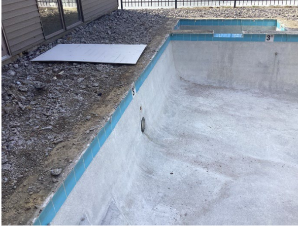
Pool plaster finish with tile perimeter
