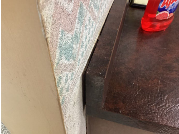
Missing sealant
