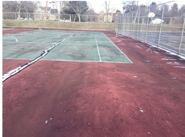
Tennis court overview
