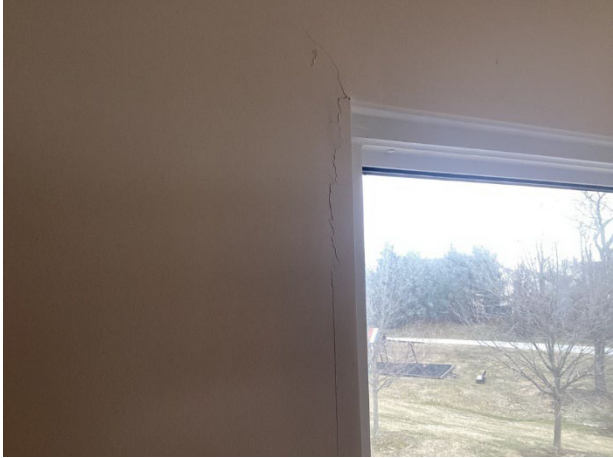
Wall crack
